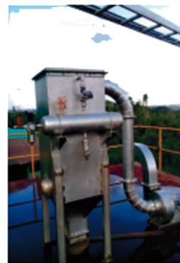
Site Location: PT. Kutai Refinery Nusantara - Plan Balikpapan - Kalimantan Timur Centralized Dust Collector - Material Transfer Process: Bottom Ash, Boiler - Power Plant
