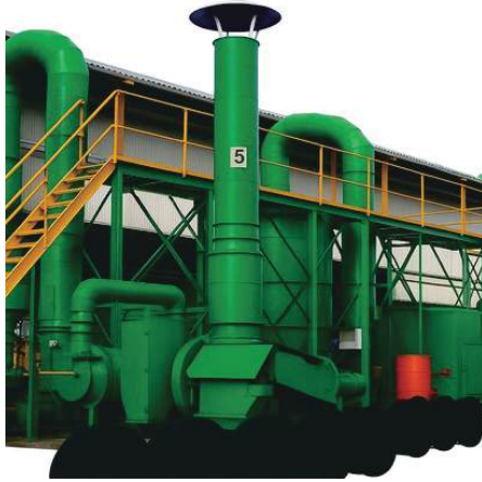
Site Location: PT. Indonesia Railways - INKA - Madiun Centralized Dust Collector & Mobile Dust Collector Sandblasting Room ( 40 x 40 x 40 ) meter; Finishing Gerbong (Sanding)
