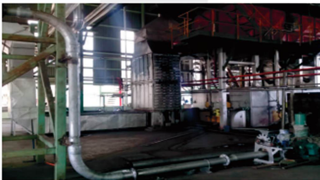
Site Location: PT. Kutai Refinery Nusantara - Plan Balikpapan - Kalimantan Timur Centralized Dust Collector - Material Transfer Process: Bottom Ash, Boiler - Power Plant
